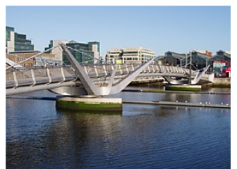
River Liffey Bridge
