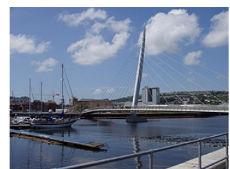
Port Tawe Footbridge
