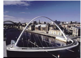
Gateshead Millennium Bridge
