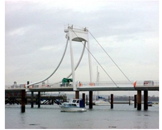
Forton Lake Bridge
