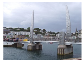
Torquay Pedestrian Footbridge
