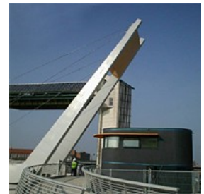
The Deep Footbridge
