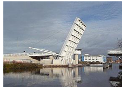
High Orchard Lift Bridge, Gloucester Quays
