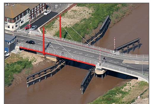
Dutch River Swing Bridge - Goole
