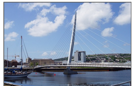
Port Tawe Bridge - Swansea
