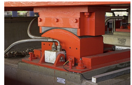
One of the seven steel/Orkot bearing blocks supporting the swing bridge
