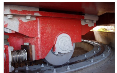
Tail wheels and main drive rack
