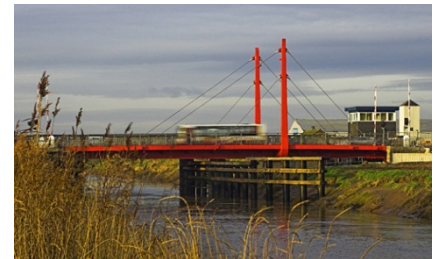
The Dutch River Swing Bridge in Goole
