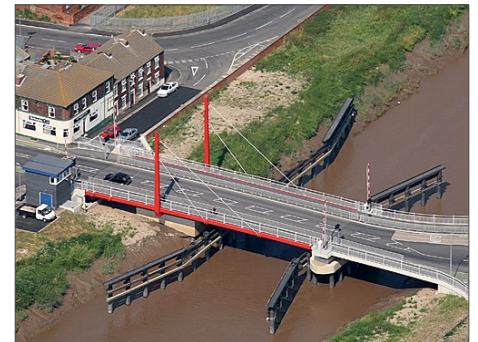
Aerial view of the Dutch River Swing Bridge
