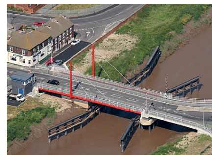
Aerial view of the Dutch River Swing Bridge
