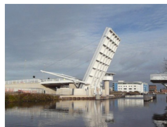
The bridge in the fully raised position
