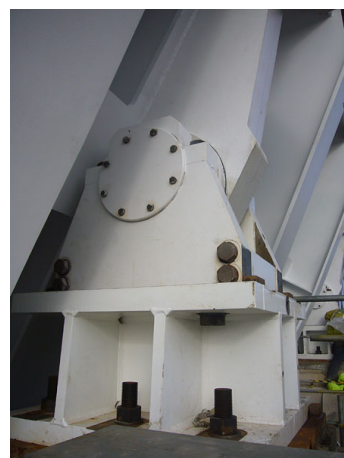
Pivot assembly and 75mm diameter holding down bolts
