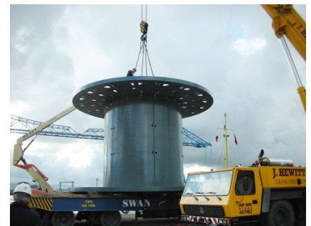
Pipe reel being lifted onto pipeline laying ship conversion
