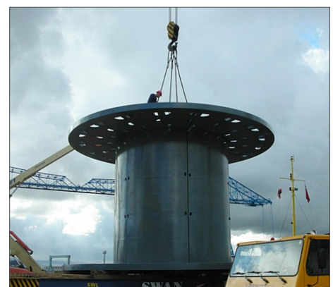
Pipe reel being lifted onto pipeline laying ship conversion
