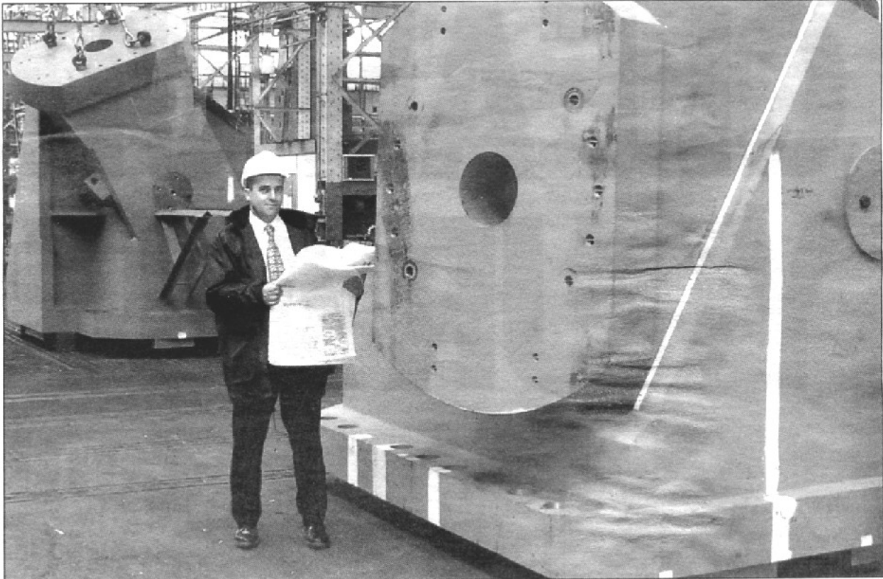
Raising the roof: Chris Carmody of Bennetts with the blocks that will carry the roof arch over the new Wembley Stadium
